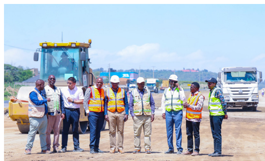
PPP committee members inspecting ongoing works at the Nairobi-Nakuru-Mau Summit highway project.
